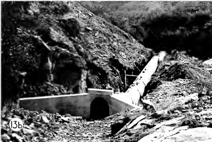
Figure 13a. Bottom Location—reinforced concrete arch on curved alignment and uniform gradient in bottom of ravine. Figure 13b. Bottom Location—reinforced concrete arch on straight alignment and broken gradient. Figure 14. Modified Bottom Location—corrugated metal pipe, with entrance in bottom of ravine and alignment following grade tour in sidehill trench, to an outlet well above and to one side of natural channel.
